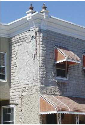
Left: Permastone and stucco cover original brick
