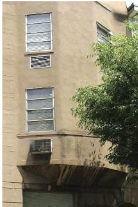
Left: Permastone and stucco cover original brick
