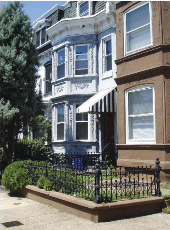
Left: Original wrought iron fence
